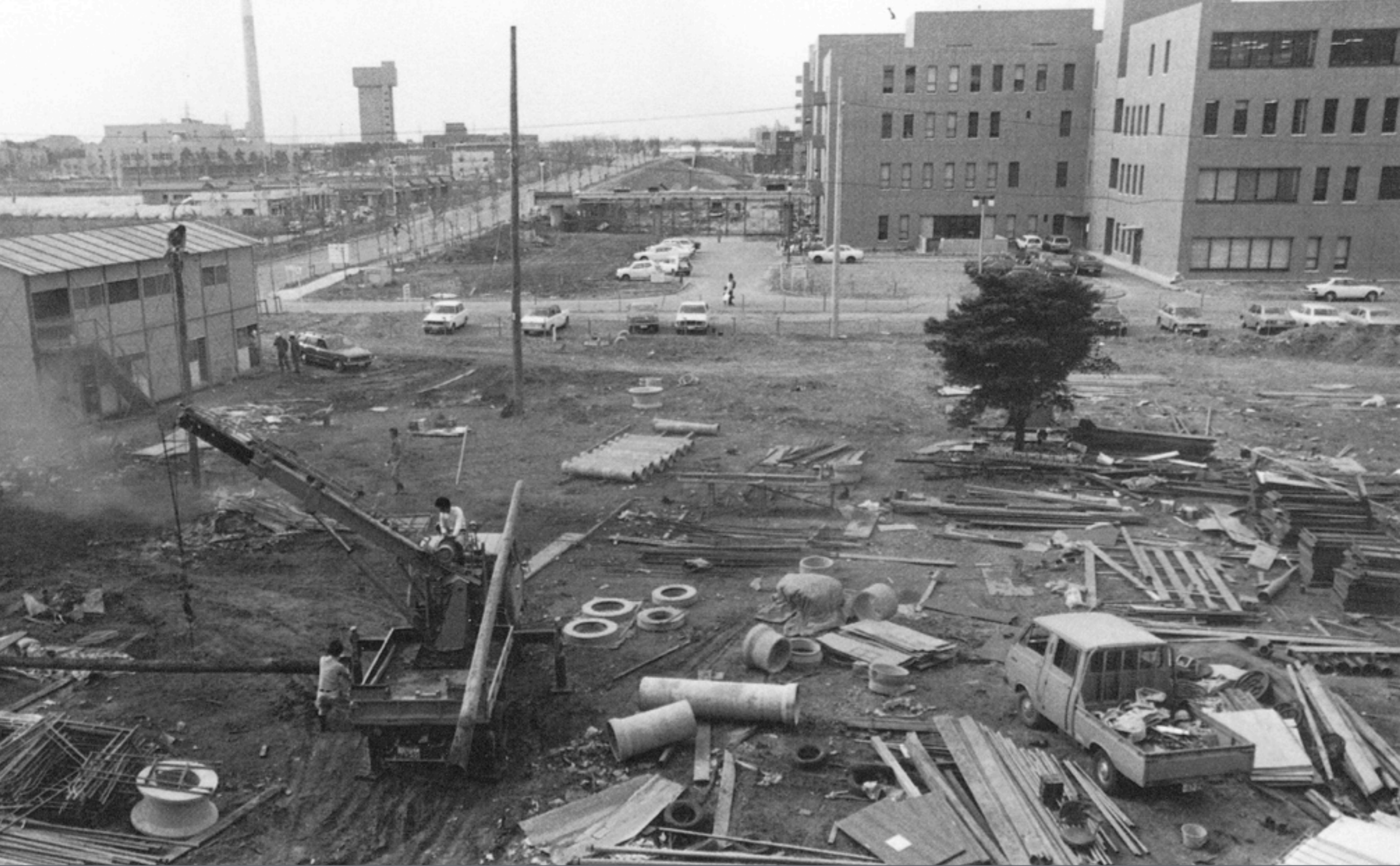
Faculty of Art and Design under construction University of Tsukuba, Early 1970s
